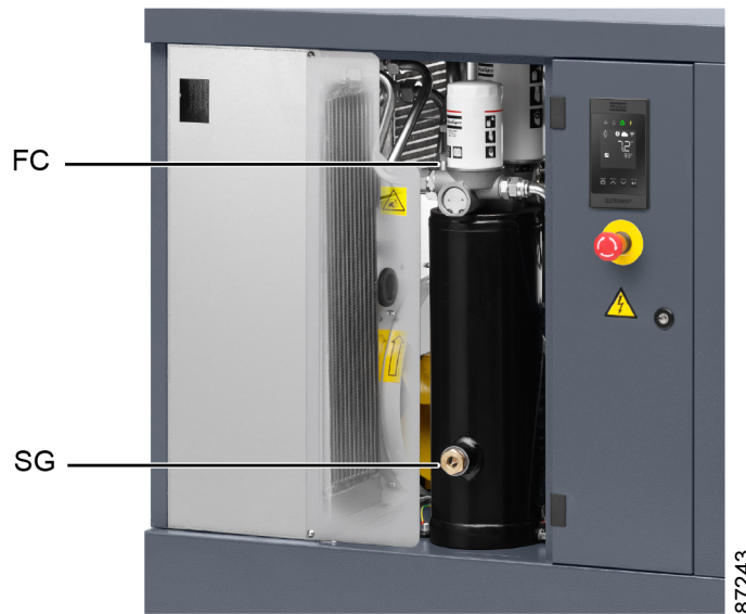
Figure 44: Oil level sight-glass
