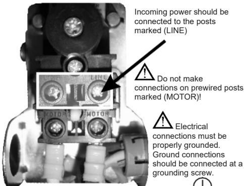
Incoming power should be connected to the posts marked (LINE)
