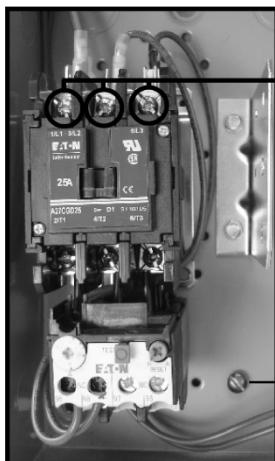
Incoming power should be connected to L1, L2 & L3 at the top of the Magnetic Starter.
